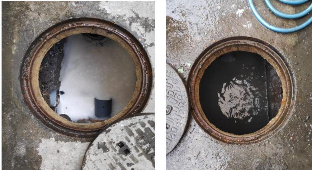
Gambar 8 Bak Collecting Tank Laundry
