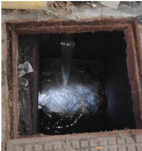
Gambar 9 Bak Collecting Tank Pre-Treatment Laundry
