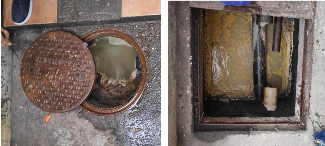
Gambar 7 Grease Trap
