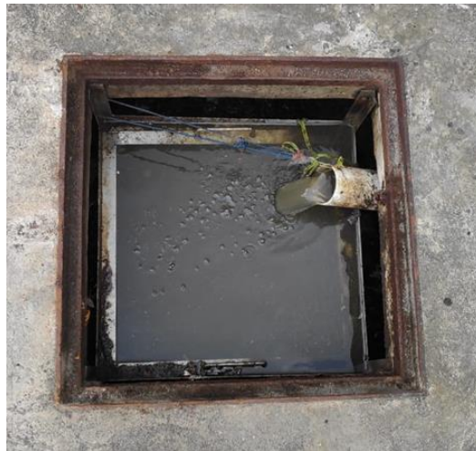
Gambar 13 Equalization Tank
