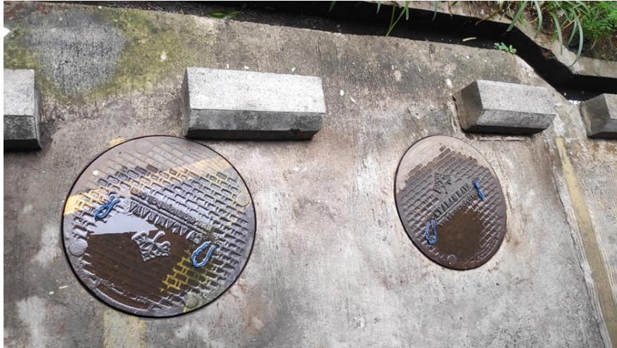
Gambar 6 Sump Pit Gedung D
